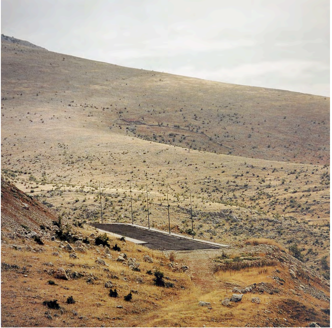
Fig. 2. G. Yerolymbos, Asphalt works, Xanthi, Thrace (from Terza Natura , 2000-3)
